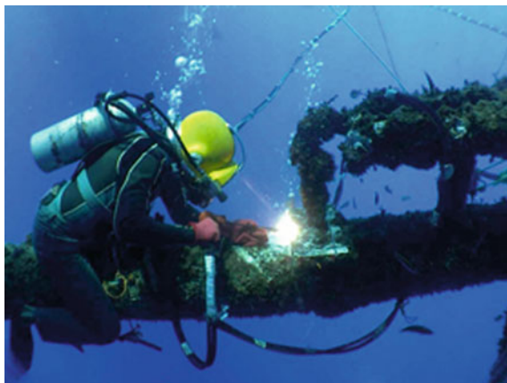
Fig. 14.10 Underwater welding ( http://underwaterweldingschools.org )
