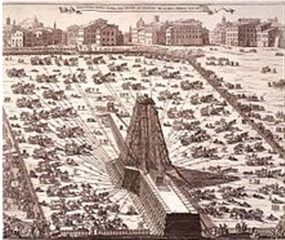
Fig. 3.10 Erection of the Vatican Obelisk in 1586 by means of a lifting tower https://en.wikipedia.org/wiki/List_of_obelisks_in_Rome
