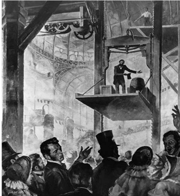
Fig. 4.14 Otis free-fall safety demonstration in 1854 (99percentinvisible.org)
